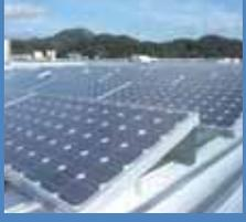
Crystalline silicon solar cells
